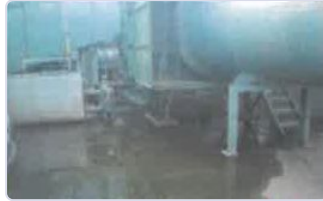
Before: condensate discharged, its energy lost
